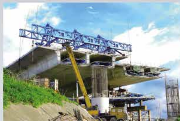
• Bridge construction Monitoring
